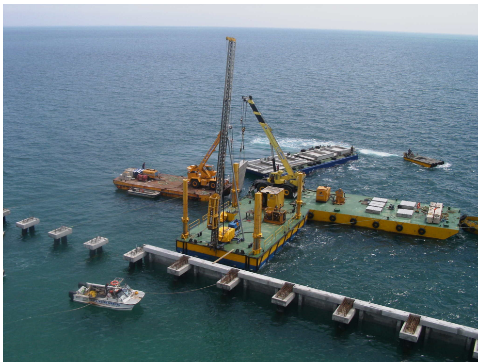
Figure 4. Construction photo showing the installation of the precast concrete panels
